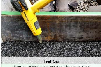
Using a heat gun to accelerate the chemical reaction can decrease curing time
